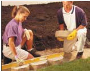
2. Place & Compact Backfill
